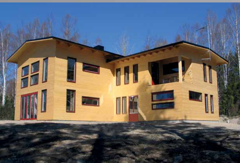
Family house built with Loglock glulam logs.
